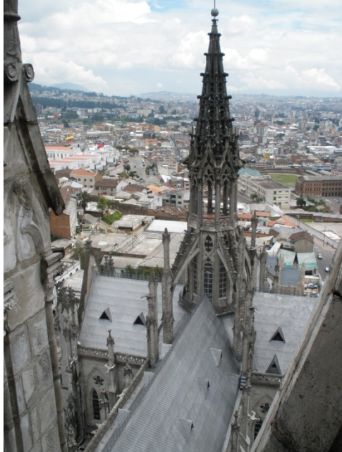
Figure 5: View from one of the towers at Basilica Del Voto Nacional
