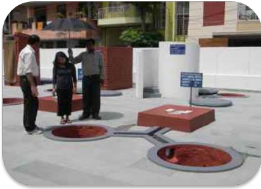
Sulabh - September 6: A Sulabh circular two-pit substructure.
